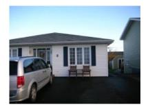
Sloped roof covering: The sloped roof cover consists of Asphalt shingles.
