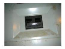
Main service voltage:120/240 volts.Location:Basement.Grounding is:Copper.
